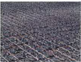
Driveway - 'noir' concrete cobbles
